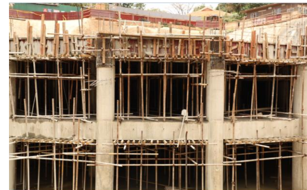
The basement that has the completed 2 nd and 3 rd floors
