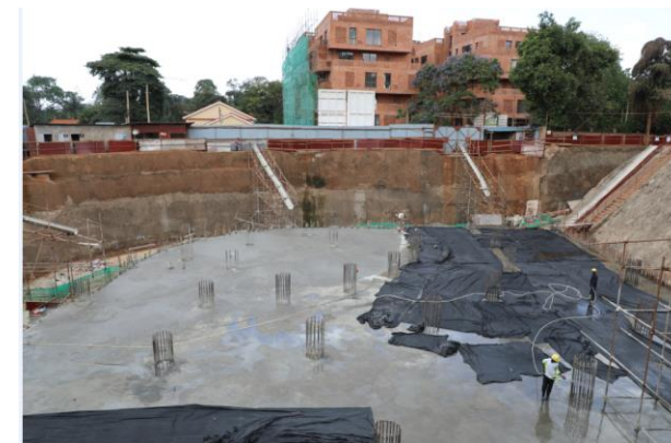
From the Top, columns that will support the 4 th basement floor.
